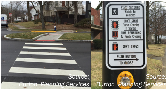
Figures 5.1-2: High-Visibility Crosswalk and Accessible Pedestrian Signal
